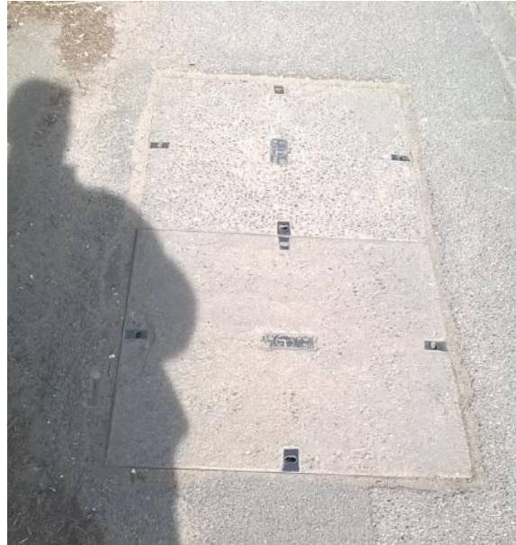
Image 5: View of existing utilities cover within footway at crossing point.
