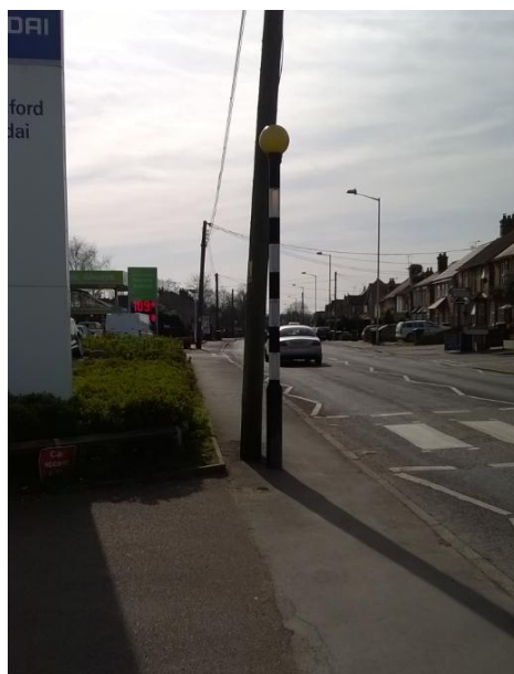
Image 3: View of existing utilities and footway width.
