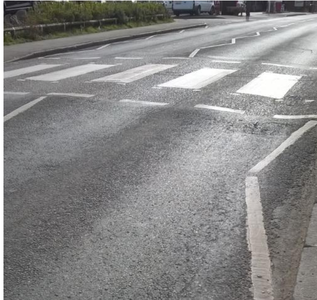
Image 6: View of rutting of existing carriageway.
