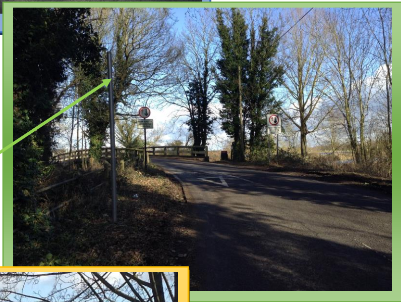
The 'Weak Bridge' sign is missing from the post at the northbound approach to the bridge
