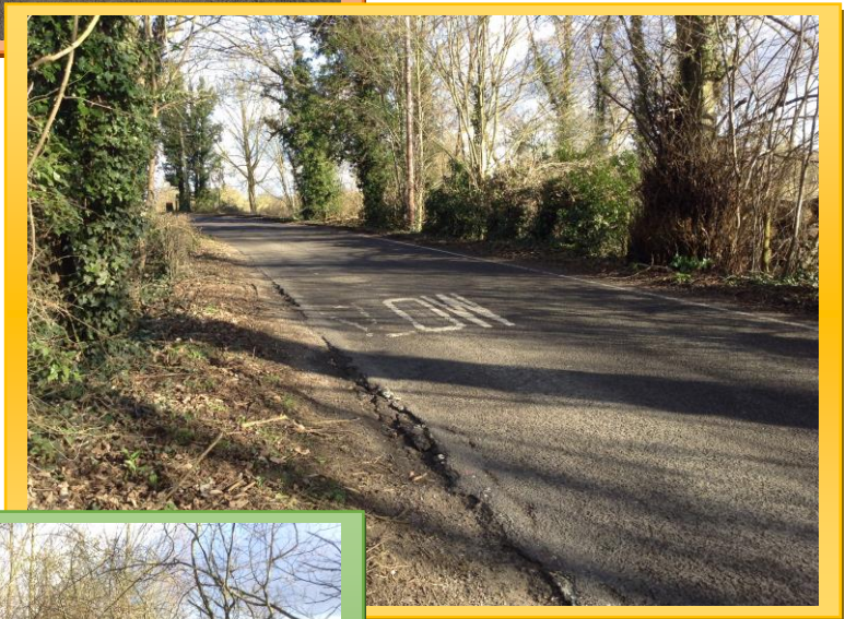
Existing road markings worn.
