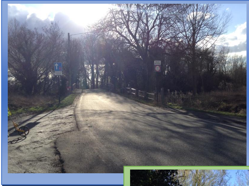
The 'Weak Bridge' signage 7.5t to TSRGD diagram 626.2A at the southbound approach to the bridge.
