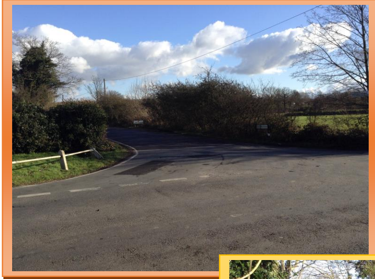
Church Road / Hammonds Road junction markings worn.
