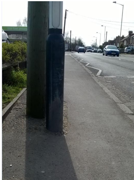
Image 2: View of existing utilities and footway width.
